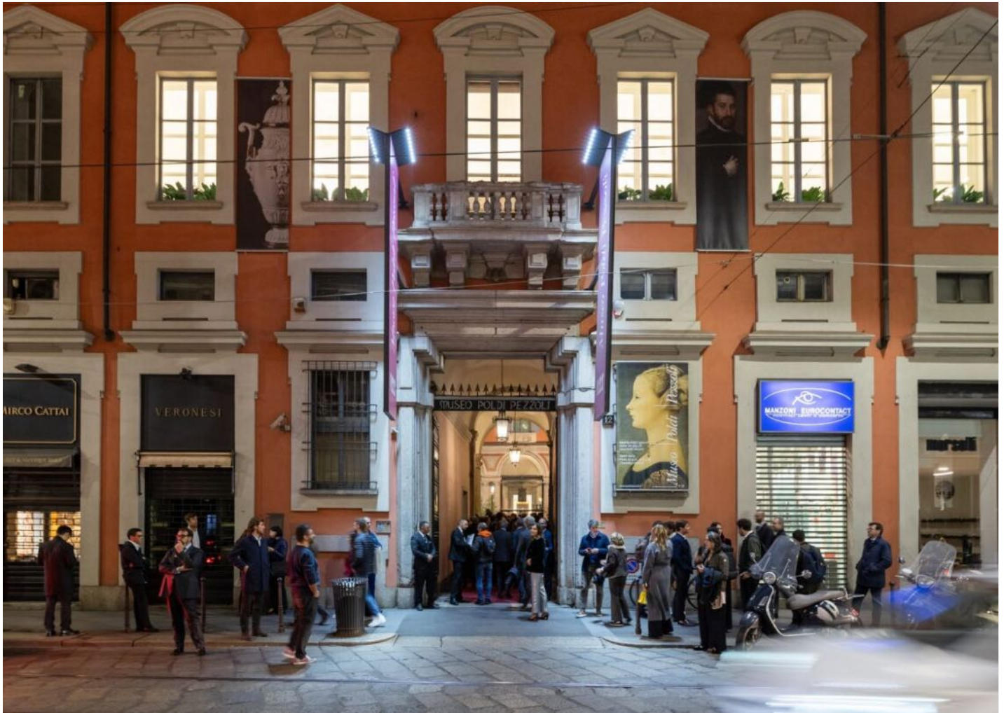
The Museum's facade. All photos courtesy of ESSECI
